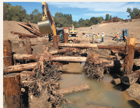
Massive logs were used to construct the riffle habitat areas.
